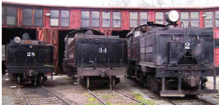
Locomotives stored at roundhouse
